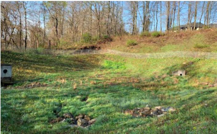
*Excess Vegetation, Ponding Water Present, Outlet Structure Obstructed*
