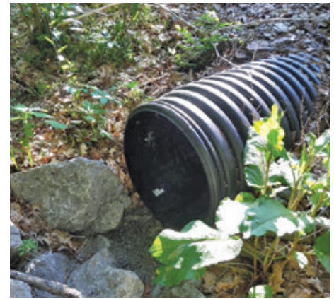
Typical storm sewer system outfall tested as part of the Illicit Discharge Detection and Elimination (IDD&E) Program (MCM #3)
